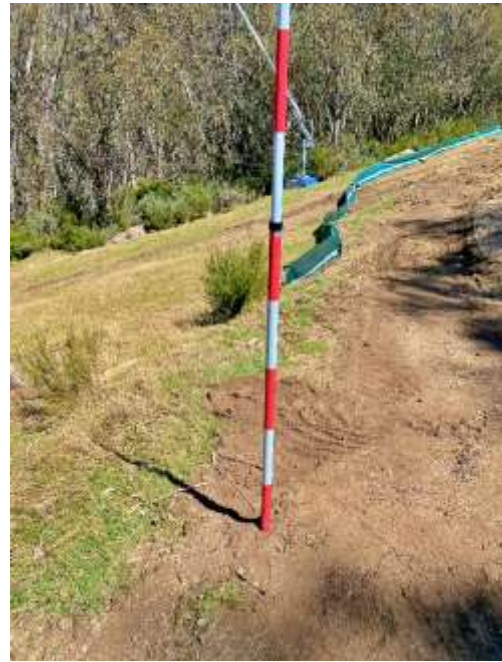
Plate 7. Slope erosion present, with erosion reduction measures installed
